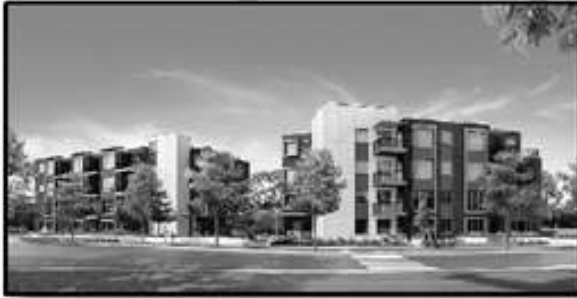
The proposed two condominium development on Borden near the Monkey Tree Pub was recently approved by Council
